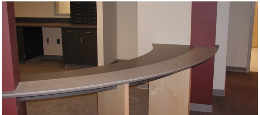
A reception area desk incorporates a solid surface ledge with wood legs and plastic laminate top.
