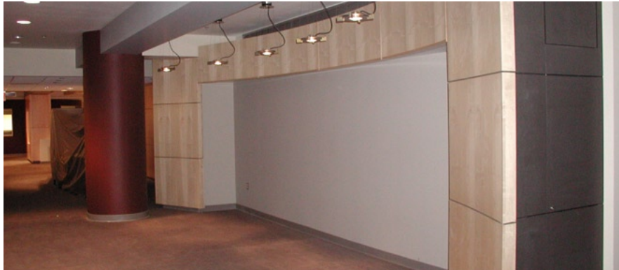
Large corridors of architecturally matched maple panels, complete with metal reveals, are a welcome addition to the typical casework.
