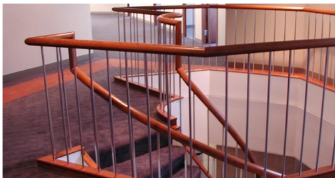
The centerpiece of the project: a chrome and red oak spiral staircase that allows the three floors to be accessed without using the public elevators
